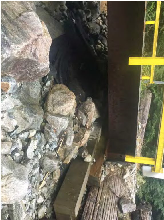
Right Bank Abutment when facing downstream
